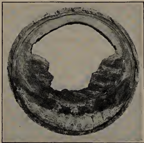
FIG. 175. Cross section of a boiler tube showing the deposit of scale
